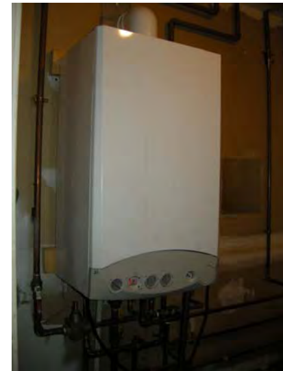
New high efficiency combination heating and domestic hot water boiler
