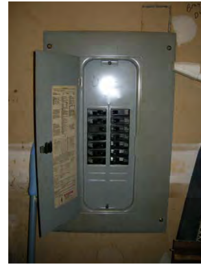
Typical circuit breaker panel
